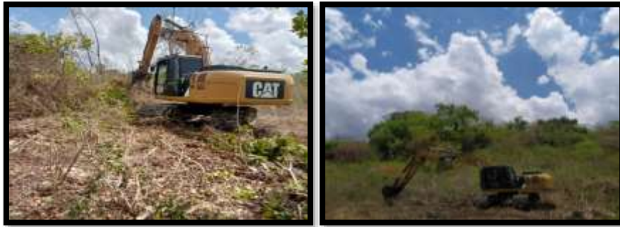
Gambar 31 Dokumentasi Sewa Excavator Pematangan Lahan Gemerlap
