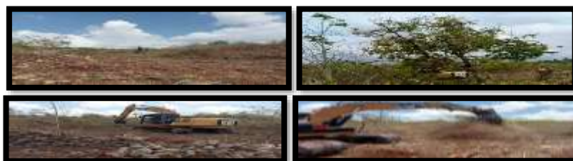
Gambar 30 Dokumentasi Sewa Excavator Pematangan Lahan Gemerlap
